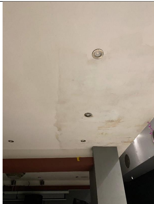
Appendix 8 – Basement Ceiling
