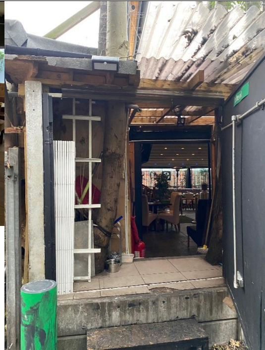
Appendix 6 – Rear fire exit
